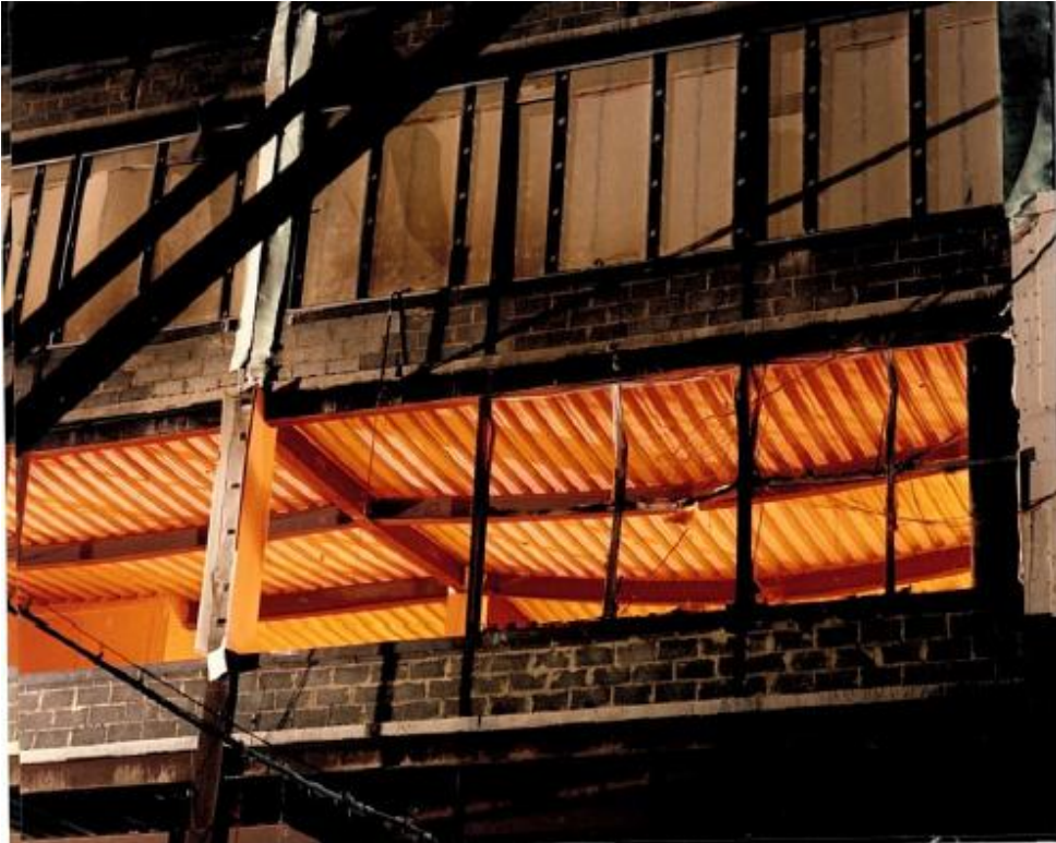
Photograph 8 Latter stages of the fire showing deflection of the secondary beams and floor slab
