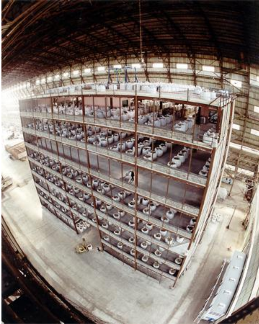
Photograph 1 Composite steel framed building inside the Large Building Test Facility at Cardington
